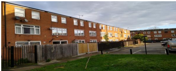
Rear of 26-42 Ashenden Road
